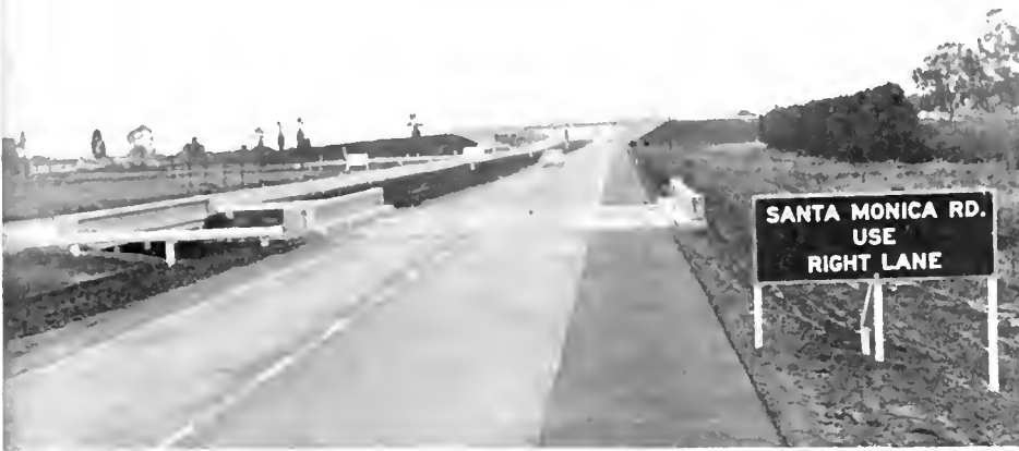
Looking west on Carpinteria Freeway. Franklin Creek Bridge in foreground and Seventh Street Overpass in background.
